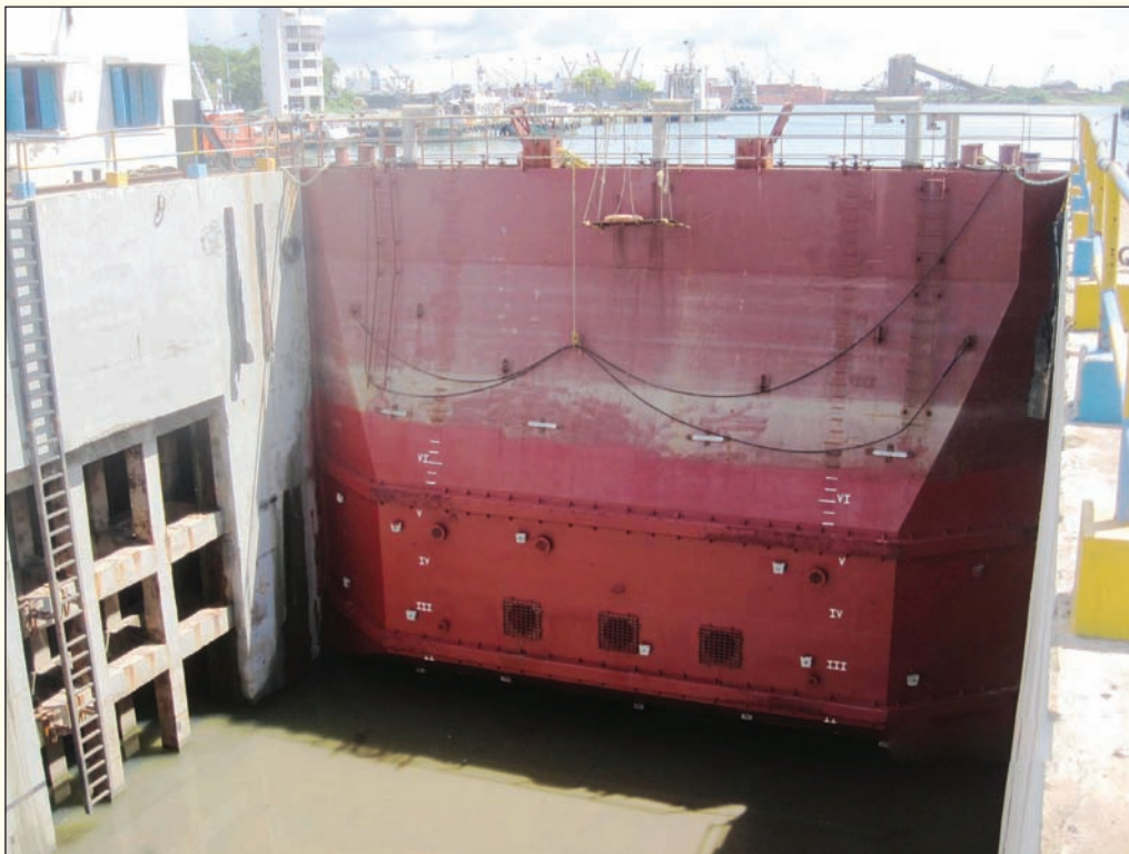
New Caisson Gate
